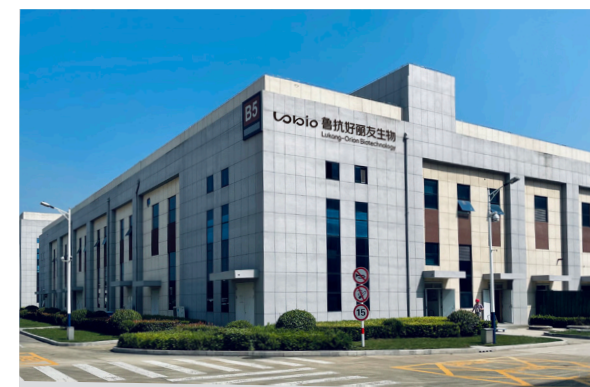
Production Facility of Lukang Hao Li You
